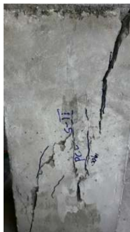
(i) Control PC column
