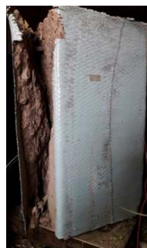
(iv) Pre-damaged and Hybrid strengthened
