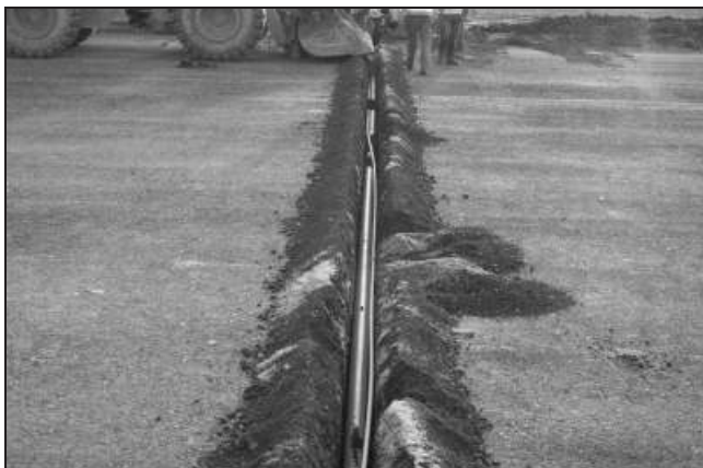
Figure 6. Typical horizontal inclinometer installation
