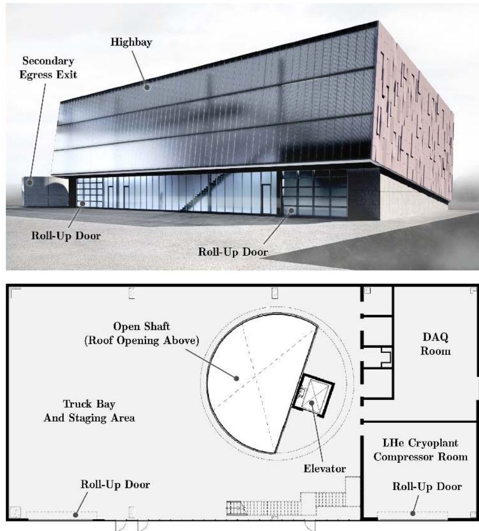
Figure 179. The Near Detector facility includes a steel-frame building located above ground and on top of the primary shaft. The front façade incorporates transparent cladding which provides a well-lit highbay for equipment staging.
